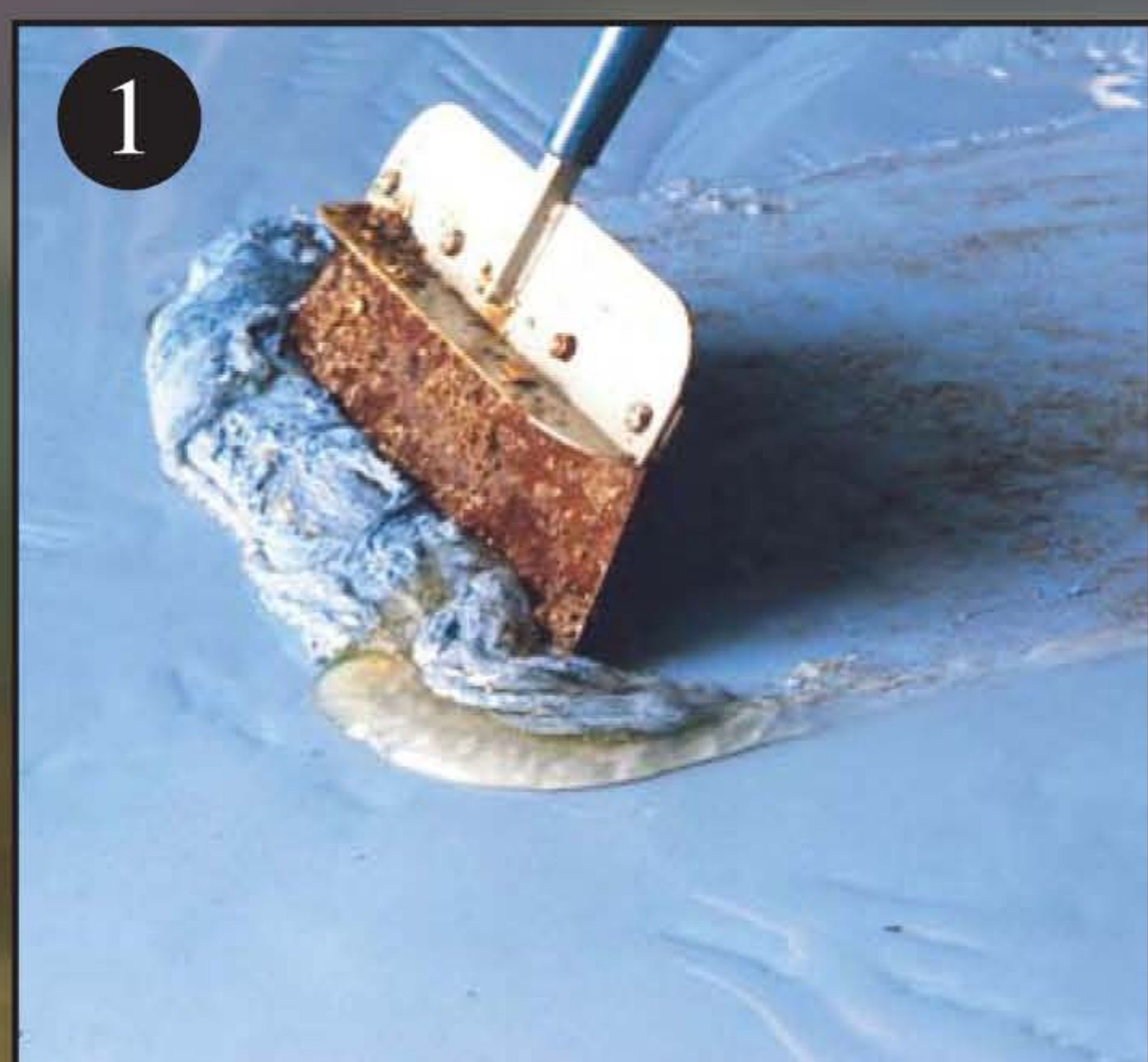
1 Scraping softened epoxy floor paint
