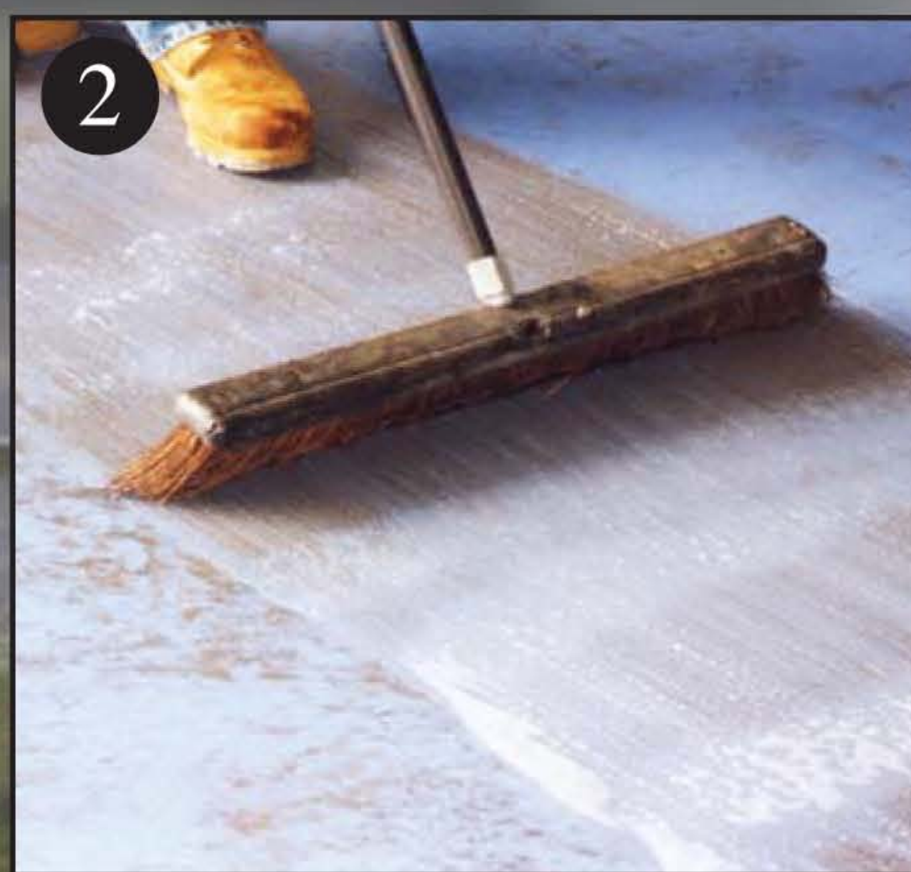
2 Scrub floor with degreaser
